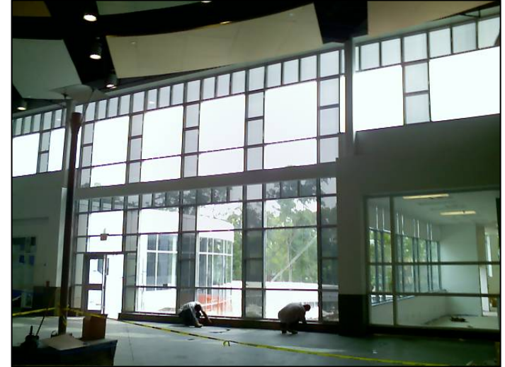
Solar Glass (Installed 2.5 KW Microsoft School of the Future, Philadelphia, PA, 2006)
